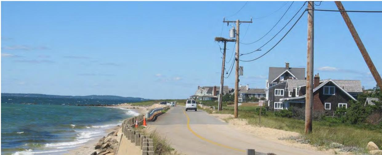
**Figure 4-19. Chapoquoit road along the barrier beach, fronted by a concrete seawall and stone revetment.**
